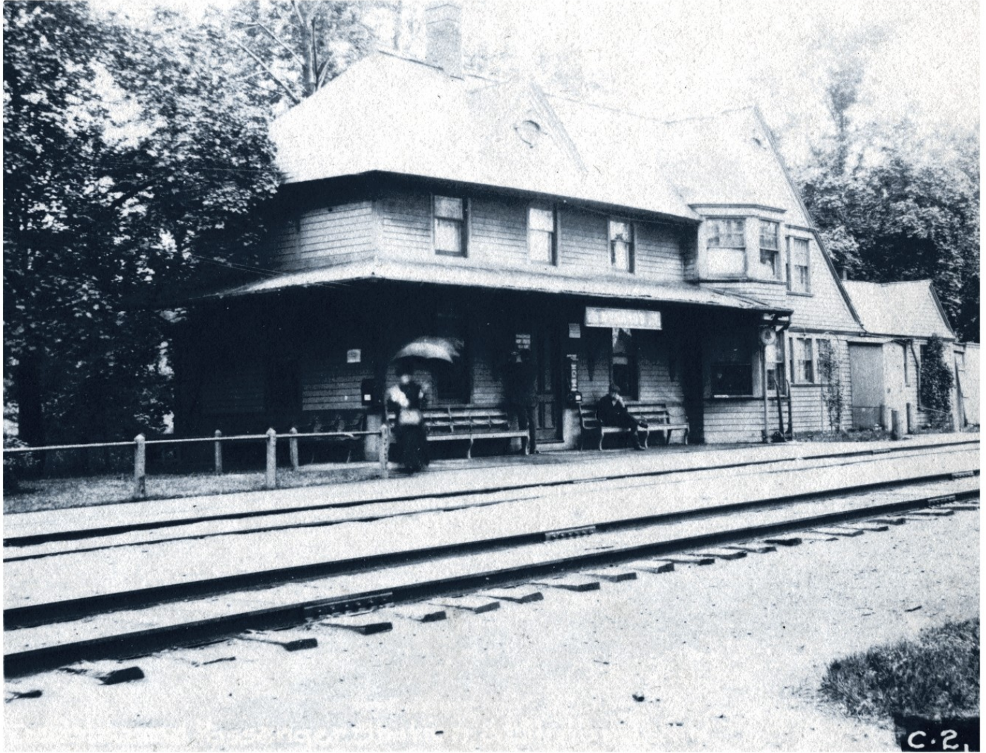
Menands Stop Railroad Station
