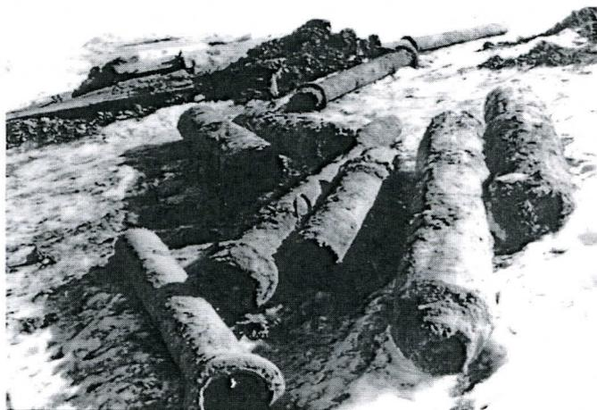
Wooden & Cast Iron Pipes of the Albany Water Works
